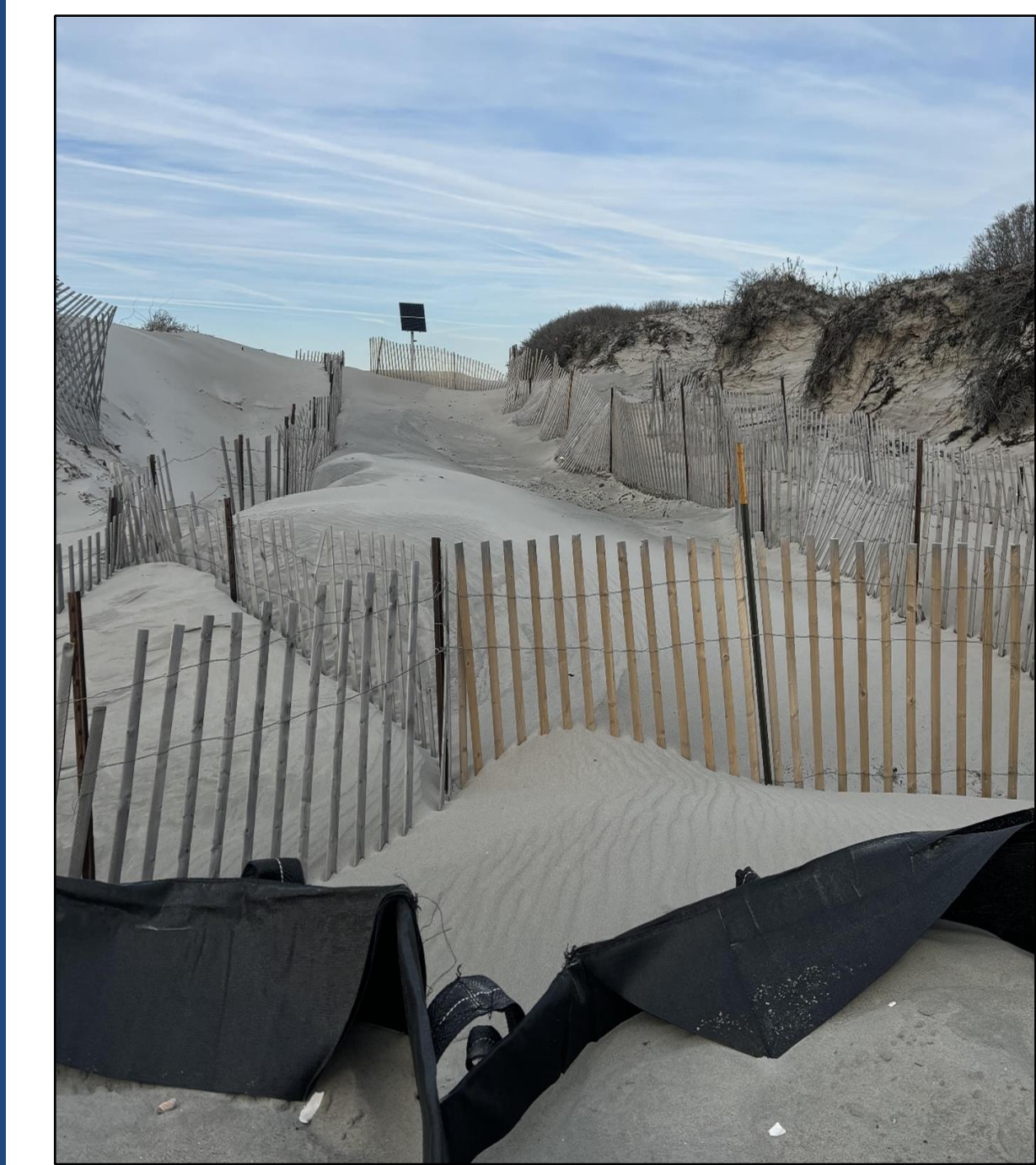
Figure 7: Dune Fencing Located At Second Beach
