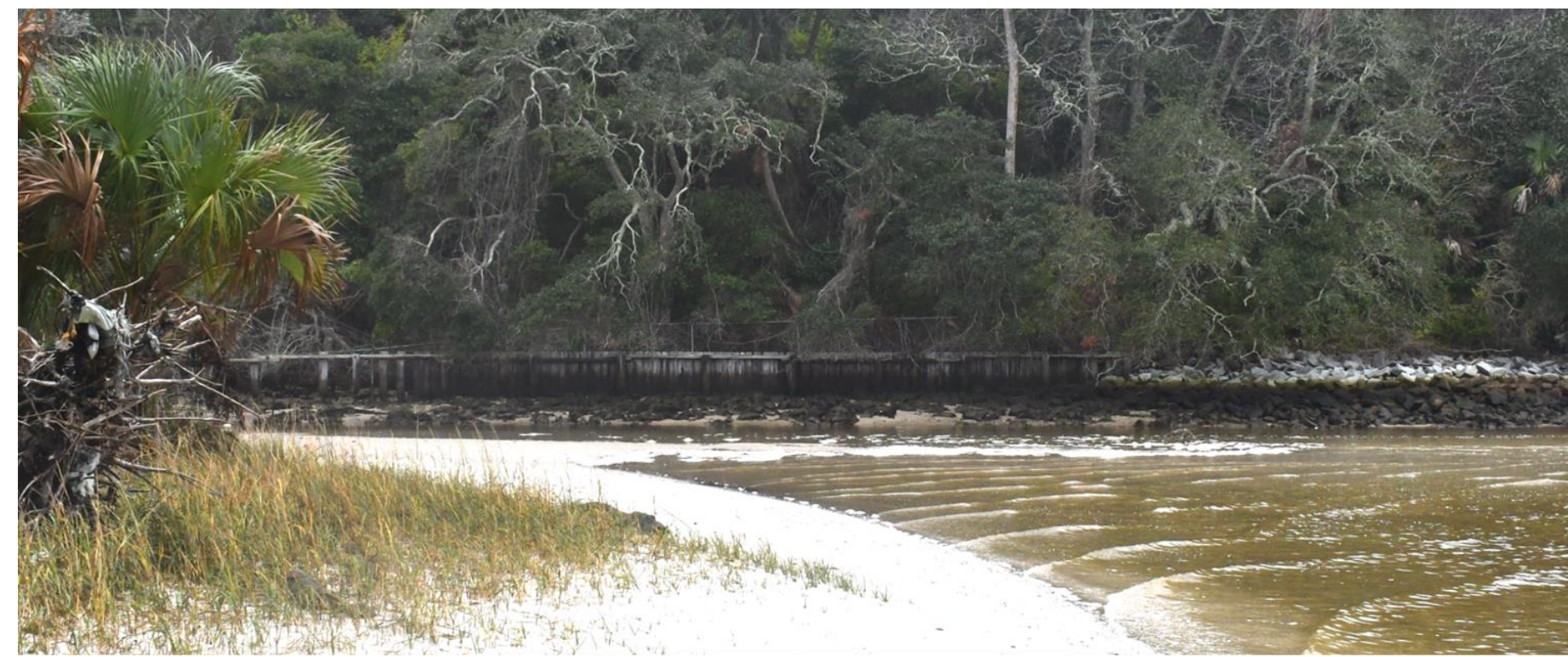
Figure 4. A picture of the current seawall (Collins)
